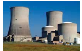
Watts Barr Nuclear Plant
